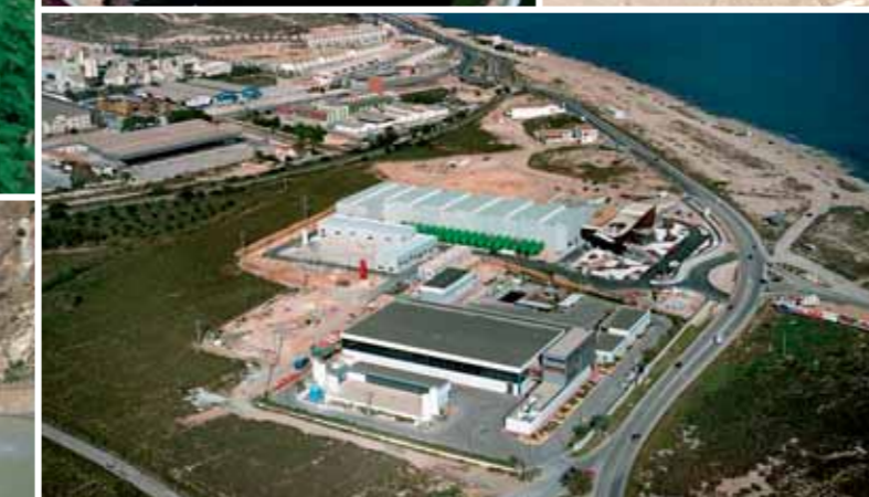
Desalination Plant Alicante (Alicante), for urban supply
