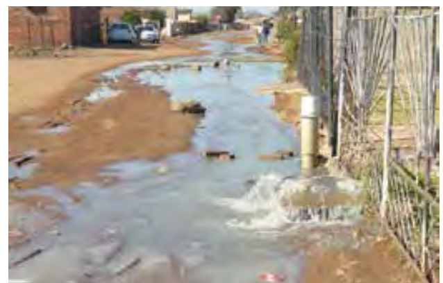
Above: Burst pipe in Evaton (© Morena Mokubung)
