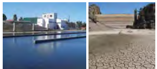
Above: Water reclamation Plant; Gamka Dam on 18 November 2011 ((© JCL Smit)
