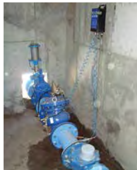
Above: Typical GSM Pressure Logger used in the Web Based data acquisition and display systems (© WRP (pty) Ltd)
