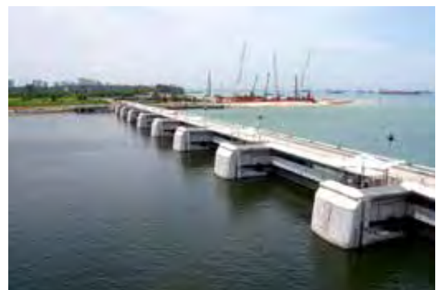
Above: The Singapore Marina Barrage creates a freshwater reservoir keeping out seawater (© ngotoh - Flickr)
