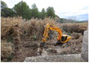
Removal of an unused weir located in the Nature 2000 Network
