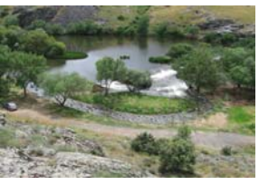
Construction of eight fish passages five of them included in the Natura 2000 Network
