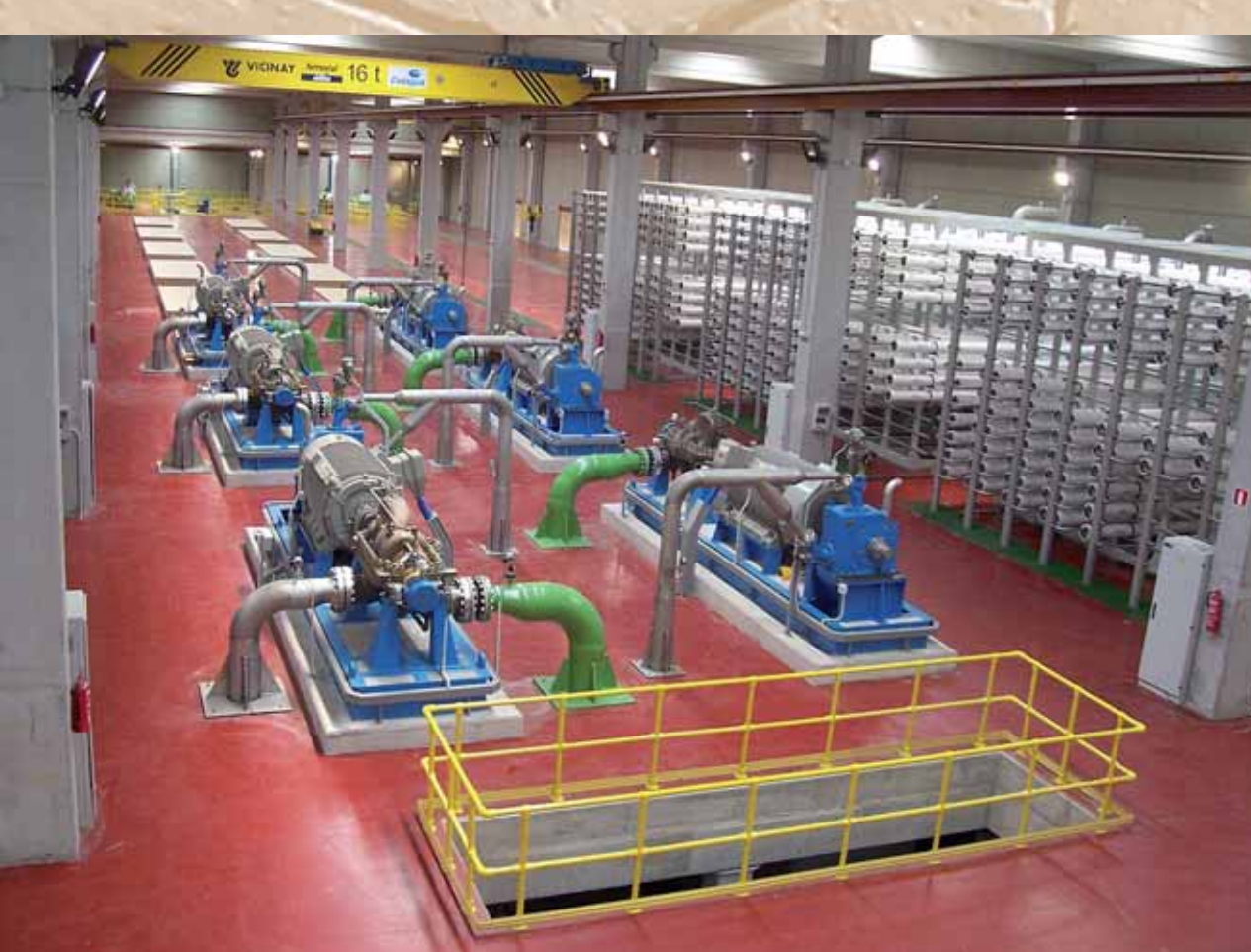
High pressure pumps and membrane racks
